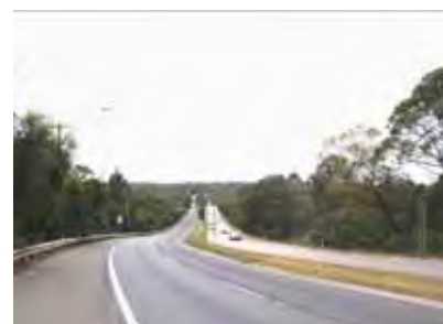
Roads present major barriers for fauna both within the site and with adjacent conservation reserves. M. Schulz/DECC
