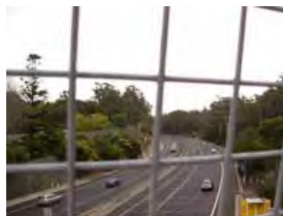
The M2 Motorway has had a significant impact on the site. M. Schulz/DECC
