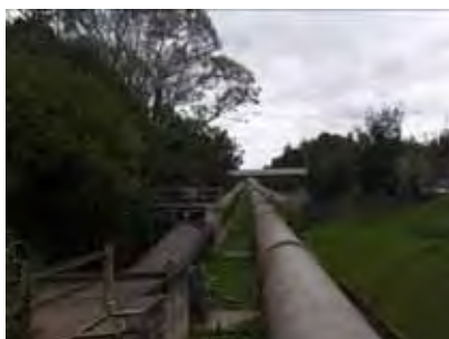
Water stored in Prospect Reservoir supplies Sydney M. Schulz/DECC
